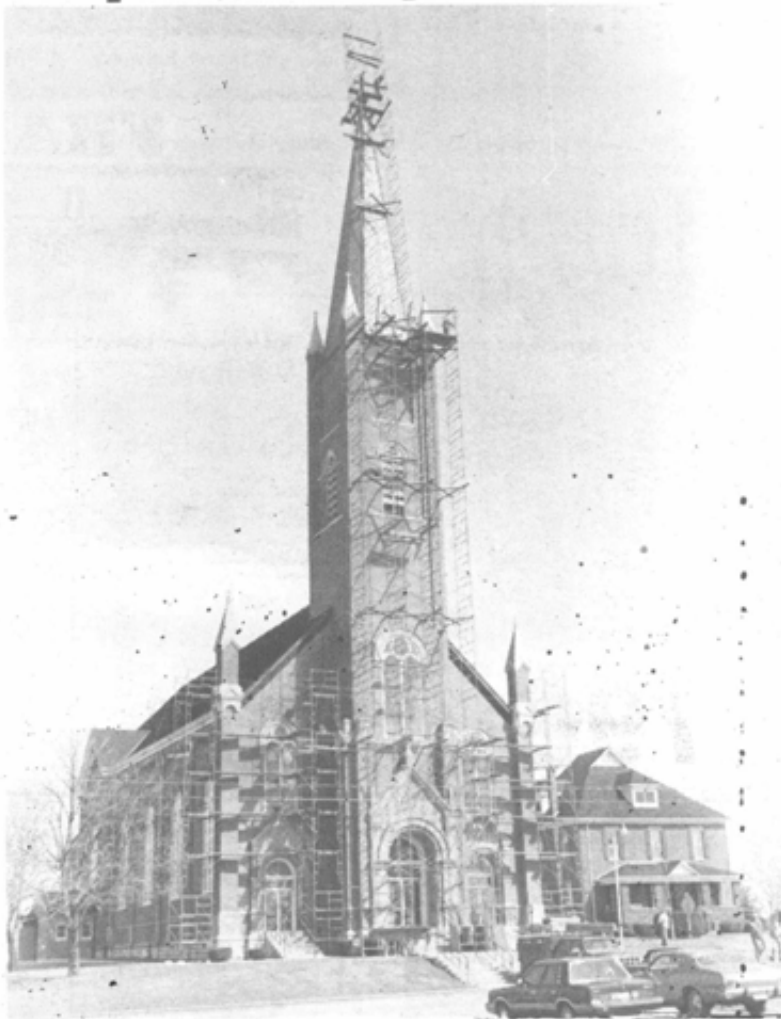
The steeple of St. John's Catholic Church in Maria Stein is under repair by Wellman Brothers in preparation for the church's 150th anniversary celebration.
